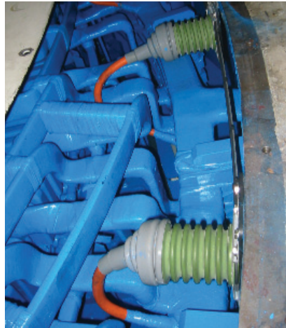
Couplers installed on a hydro generator stator
