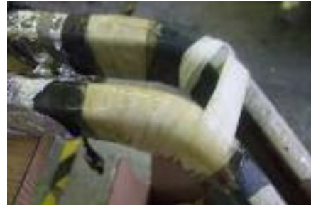
Completed insulation repair, awaiting application of the semi-con and grading coatings.
